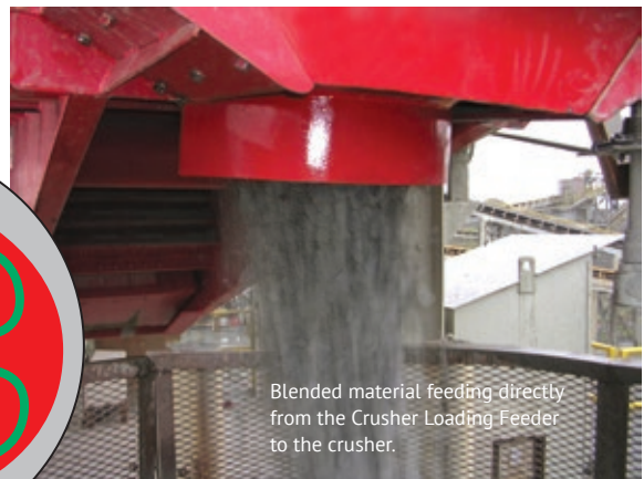
4-inch rock being distributed through the peripheral discharge of the Crusher Loading Feeder.
